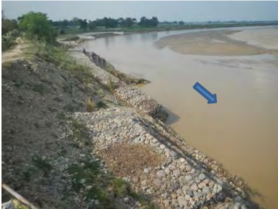
Fig.2 Revetment made of gabions①
