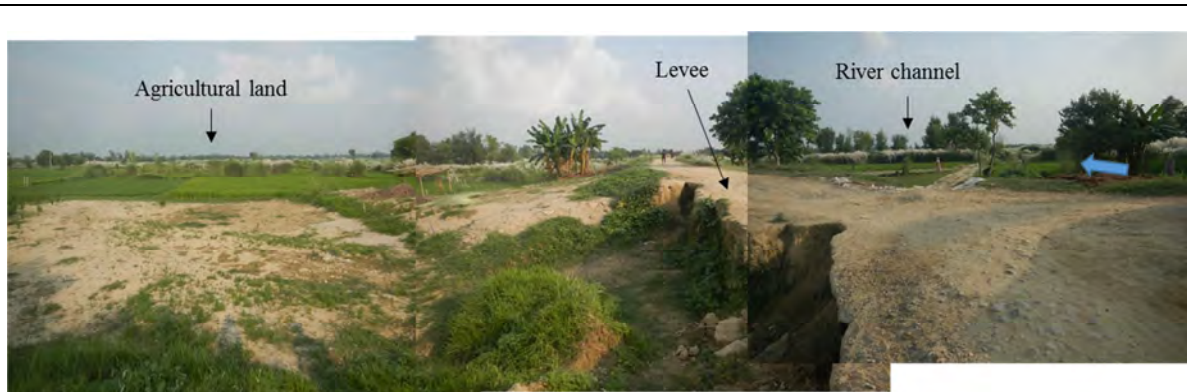
Fig.12 River channel raised by sedimentation from surrounding farmland
