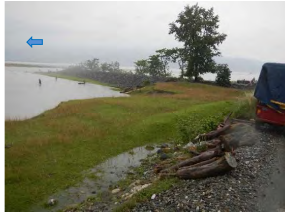
Fig.23 Spur dikes installed on the riverbank②
