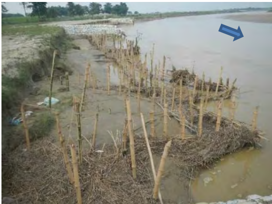
Fig.4 Bamboos and fascine set between spurs dikes
