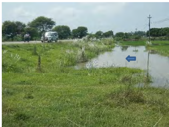
Fig.9 Drainage inhibition by road embankment①
