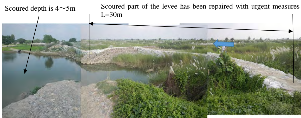
Fig.6 Lower left bank embankment under repair
