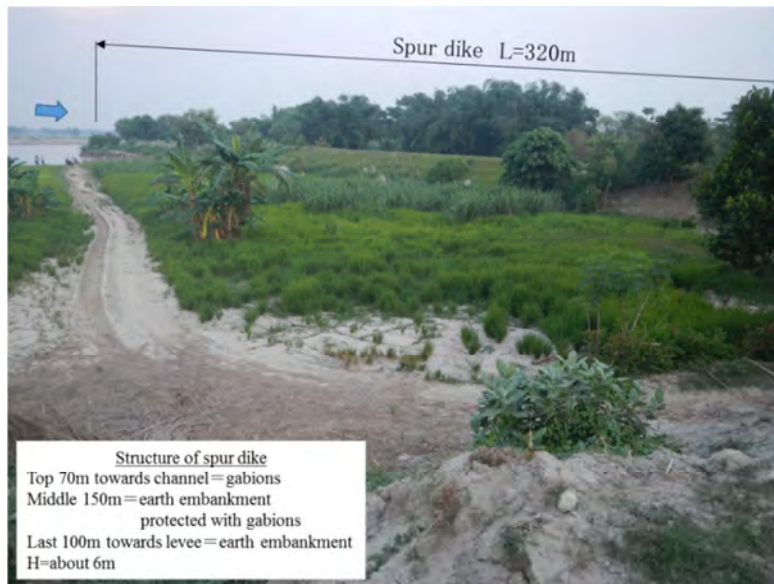
Fig.14 Spur dike built on the right bank of the river
