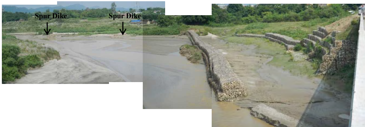
Fig.18 Double-walled revetment with gabions and spur dikes with gabions
