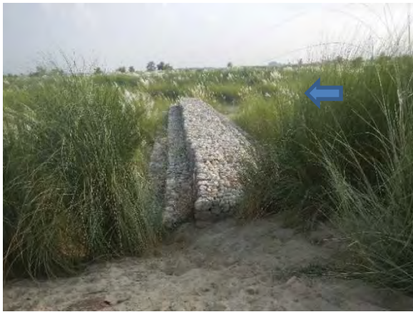
Fig.7 Spur dikes made of gabions① Spur dike made of gabions has installed upper stream of the scoured part.
