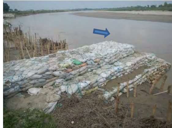
Fig.3 Spurs dikes made of sand bags and covered with nets
