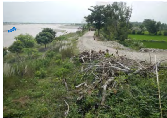
Fig.17 Raised riverbed The riverbed (left in Fig.17) is higher than the farm land (right in Fig.17).
