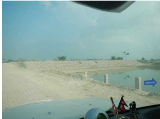
Fig.5 Revetment made of gabions②
