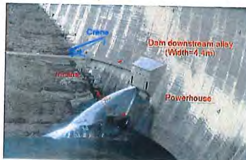
Fig. 2.2.4.5-1 Method by installing crane and incline.
