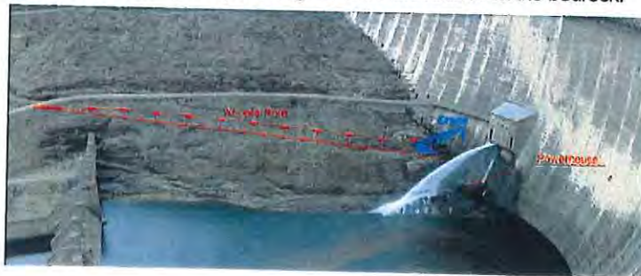
Fig. 2.2.4.5-2 Installation of access road.
