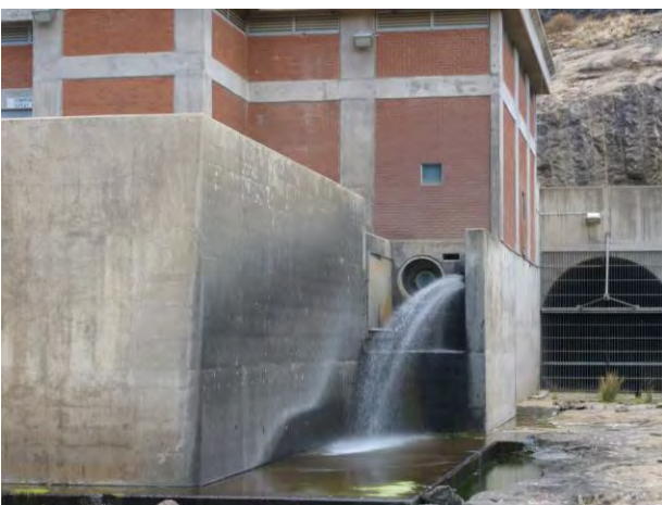
Mohale dam discharge
