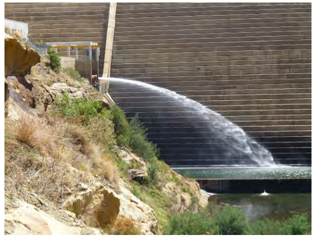
Metolong dam discharge
