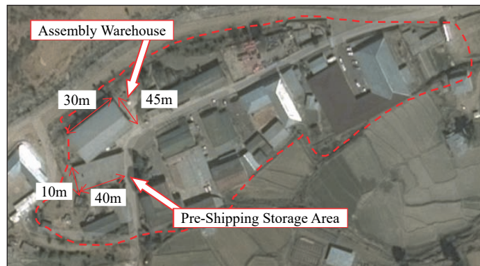
Figure 2-4: FMCL Site in Paro
