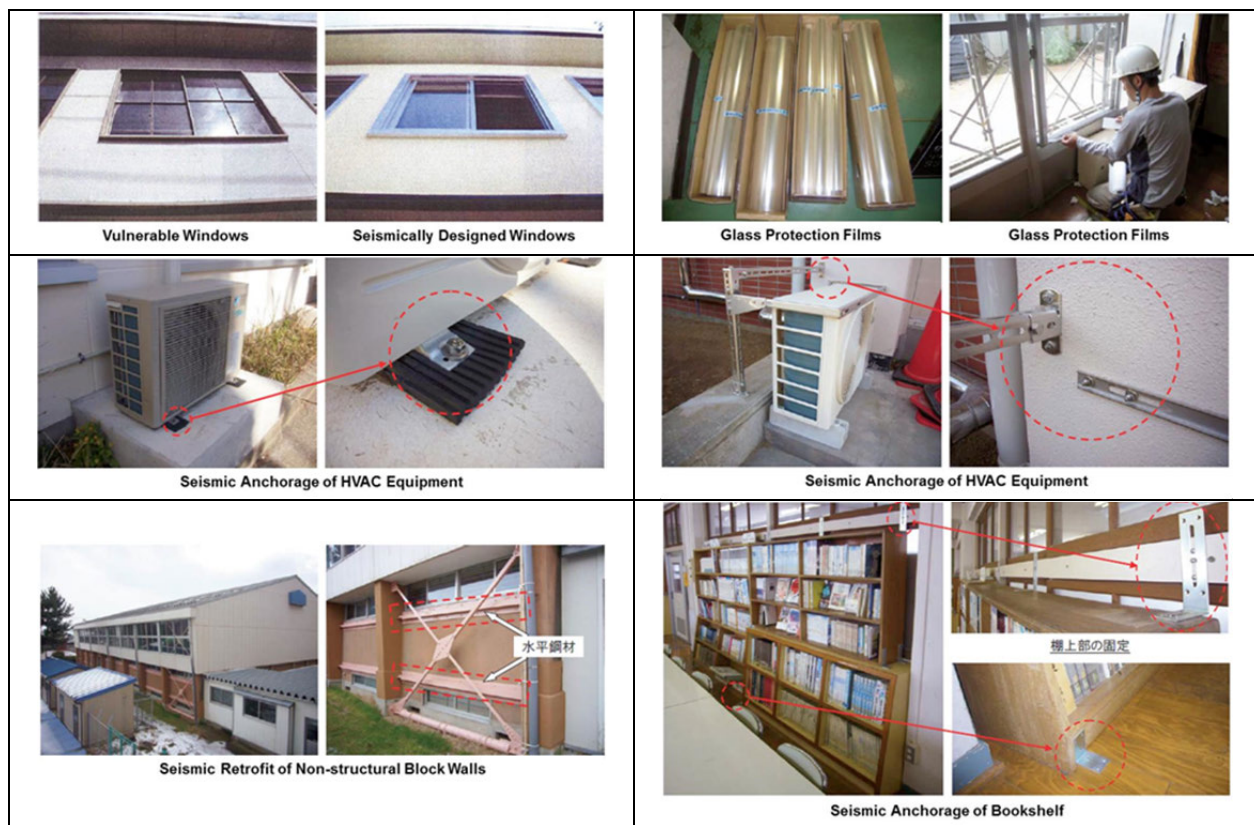
Source: Examples of Seismic Resilient Measures for Non-Structural Elements of School Facilities (MEXT)
