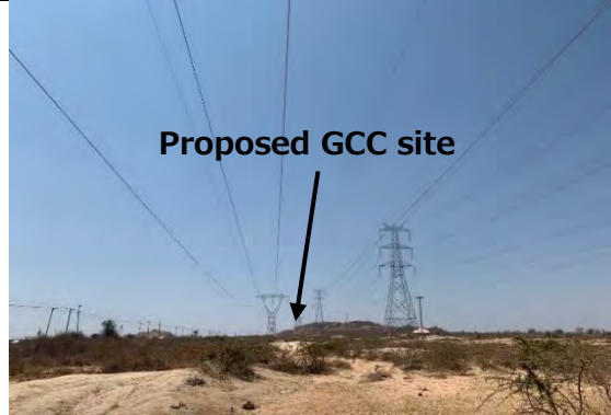
New GCC Construction Site
