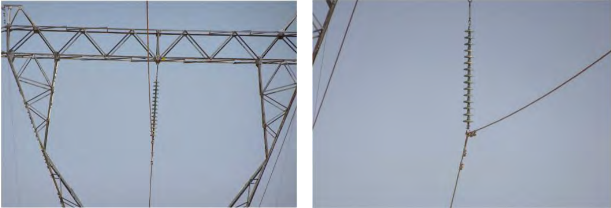
Figure 3-4.4 Status of top of existing 220kV single circuit transmission line (no arcing horns)
