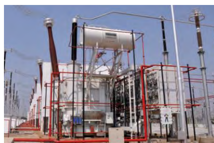
Figure 5-4.4 765 kV Class Power Transformer
