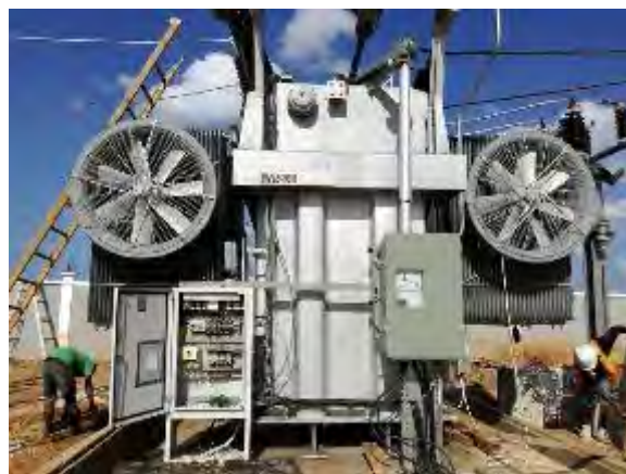
132/33kV transformer (20MVA)
