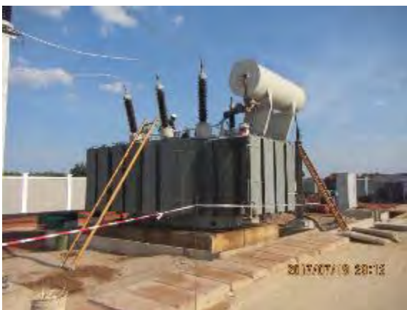
132/33kV transformer (20MVA)
