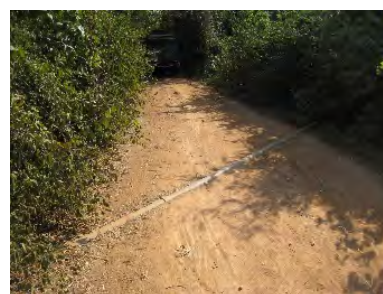
Exposed Water pipe
