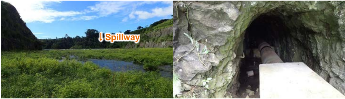
Overflow of the surplus water from the spill way
