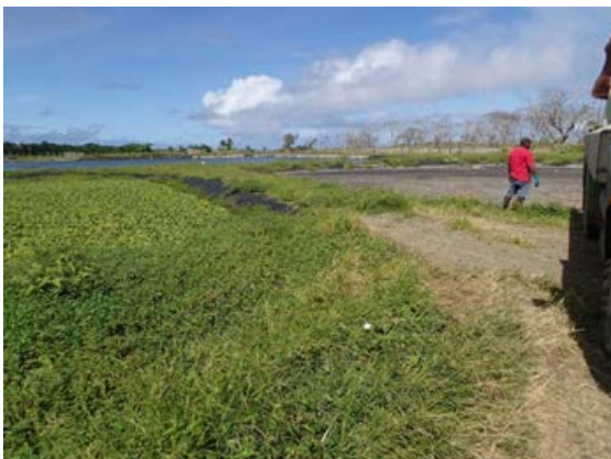
Anaerobic pond-2 (The surface of the pond is covered by grass. It is better for preventing bad odor.)
