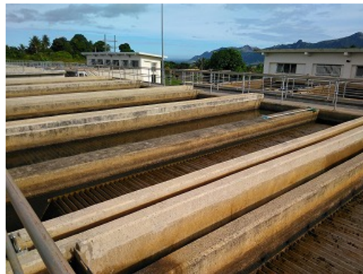
Condition of inclined plane sedimentation basin
