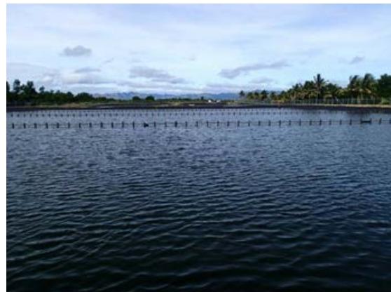
Maturation pond (Buffer piles are set.)
