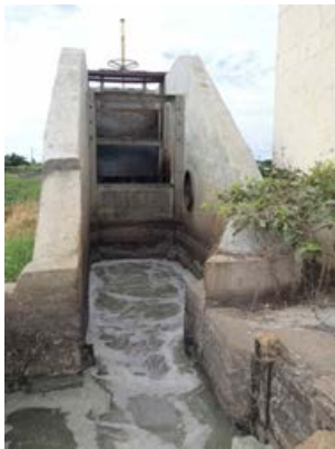
Inlet into WWTP (Wastewater is pumped from the pumping station in the city center)
