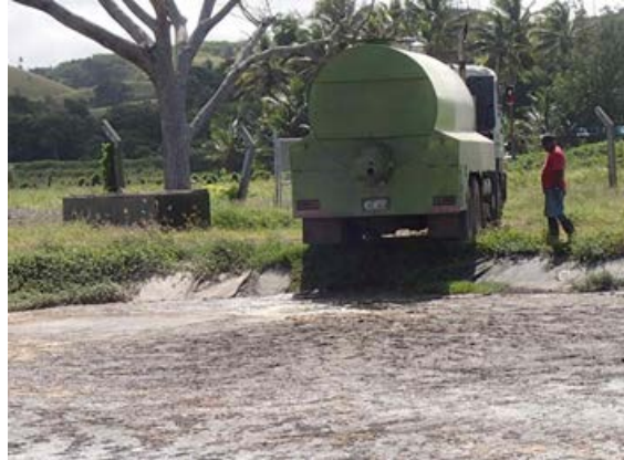
Anaerobic pond-1 (Septic tank sludge is dumped into the pond.)
