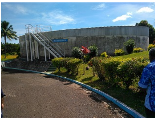
Condition of distribution reservoir
