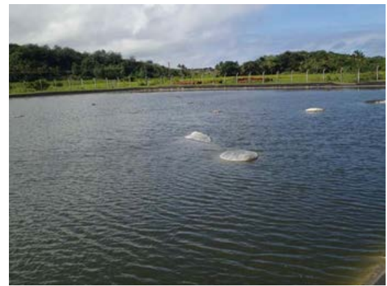
Maturation pond (A part of rubber sheet is peeled off and floats onto the surface of pond.)
