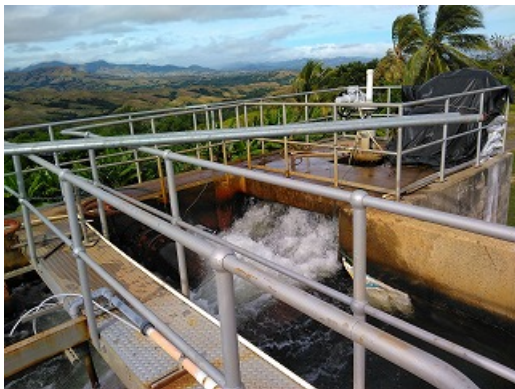
Condition of receiving well
