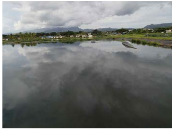
Anaerobic pond (A part of rubber sheet is peeled off and floats onto the surface of pond.)
