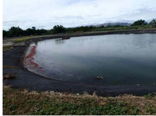
Anaerobic pond (No strong odor)
