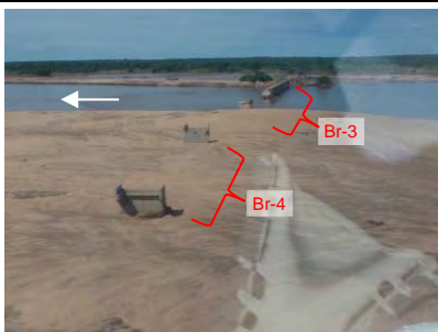
Br-4 (Licungo III): Portions except abutments were washed away and embankment between Br-3 and Br-4 was also washed away
