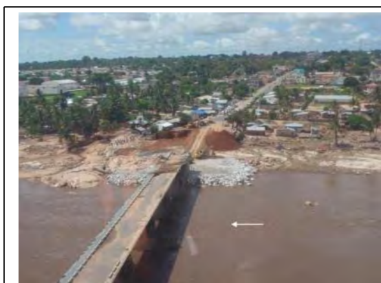
Licungo R. Br: Embankment work was started at eroded right bank.
