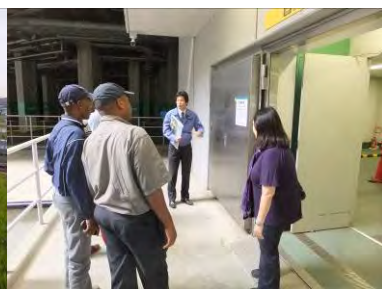
Watertight door on the building in retarding basin
