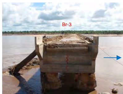
Br-3 (Licungo II): Abutment on right bank side
