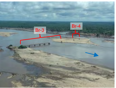
Br-3: 6 spans of right bank side are remained but beams and piers of other 3 (?) spans were washed away
