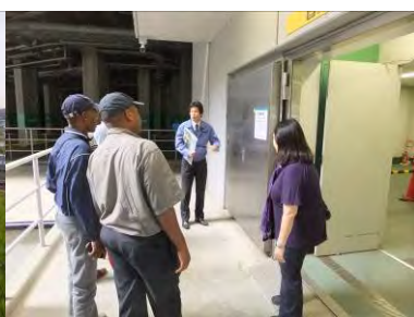
Watertight door on the building in retarding basin
