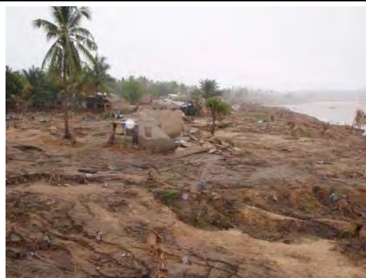
Right bank of Lugela R. at the bridge: Some houses were destroyed due to flood flow.
