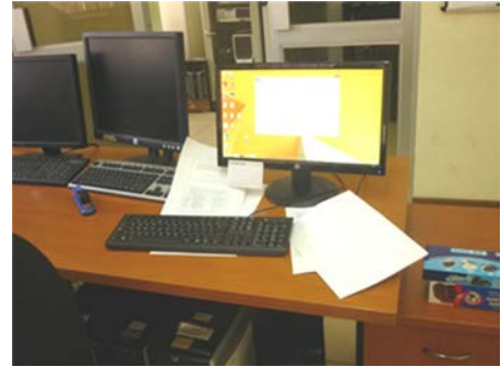
Fig. 3-18 Data storage PC
