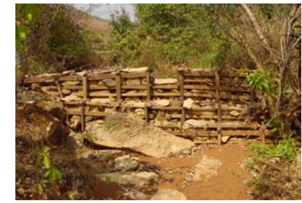
Constructing small check dams
