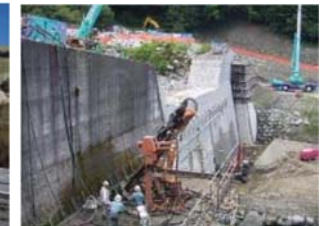
Reinforcement of sabo dam
