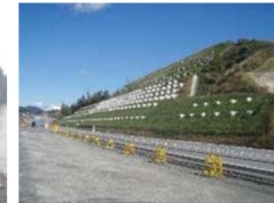
Construction to highway slopes
