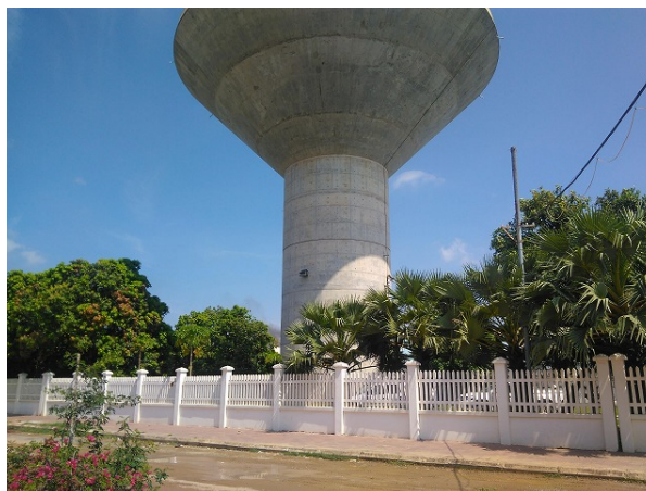
Ta Khmau Elevated Tank r
