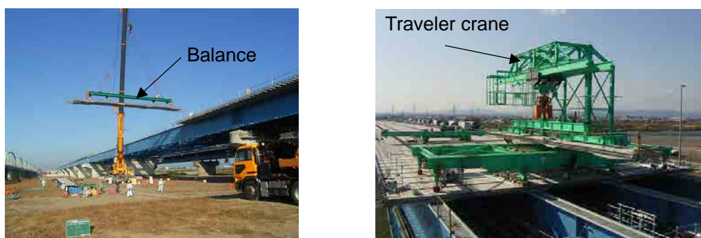
Figure 12-3-3. Construction Work by Crane (Left Side) and Construction Work by Traveler Crane on Girders (Right Side)
