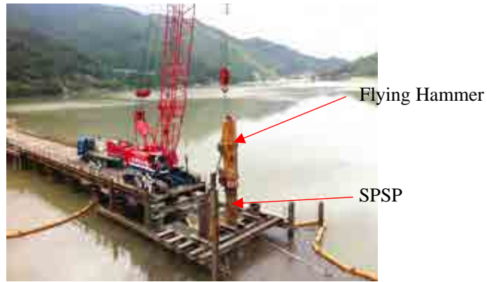
Figure 11-2-7. Flying Hammer Construction Method
