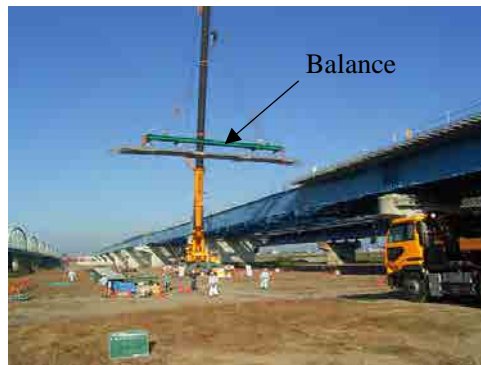
Figure 11-2-22. Reference Drawing of Hoisting Work
