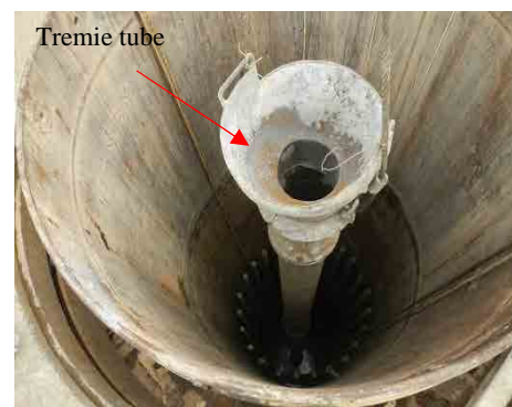
Figure 11-2-15. Reference Drawing for Construction of Cast-in-Place Pile (Placing Concrete)
