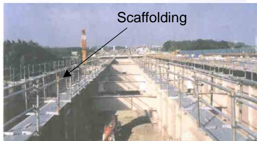
Figure 12-3-5. Scaffolding on the Steel Girders
