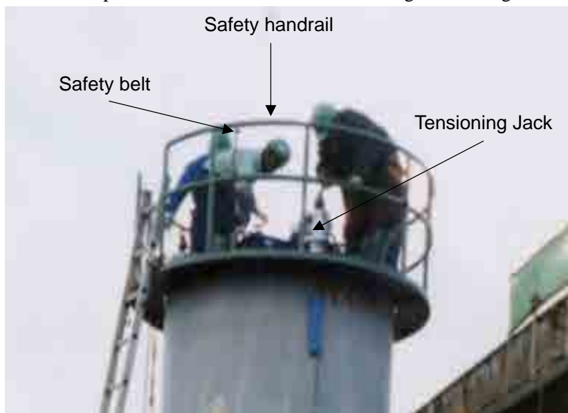
Figure 12-3-2. Tension work
