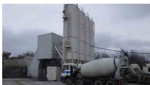
Concrete plant, Cement silo, Agitator truck
