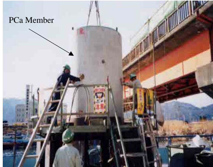
図 12-3-1. Installation of PCa member
