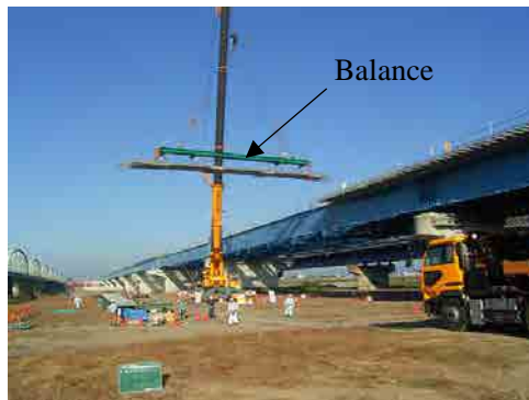
Figure 11-2-22. Reference Drawing of Hoisting Work
