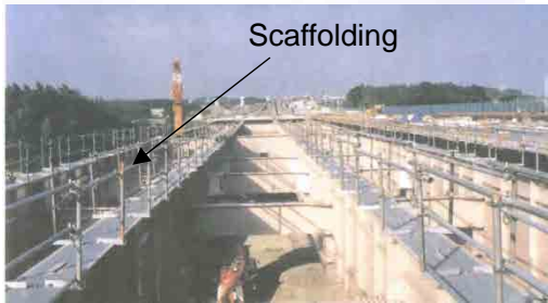
Figure 12-3-5. Scaffolding on the Steel Girders
