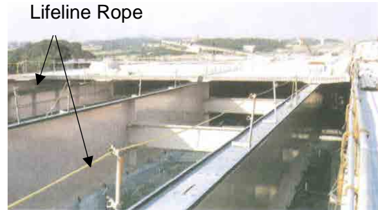
Figure 12-3-6. Lifeline Rope for Construction Work
