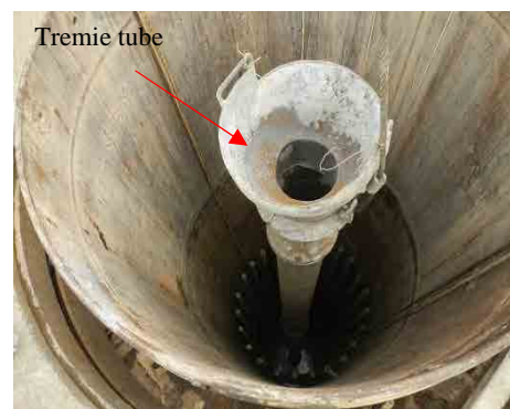
Figure 11-2-15. Reference Drawing for Construction of Cast-in-Place Pile (Placing Concrete)
