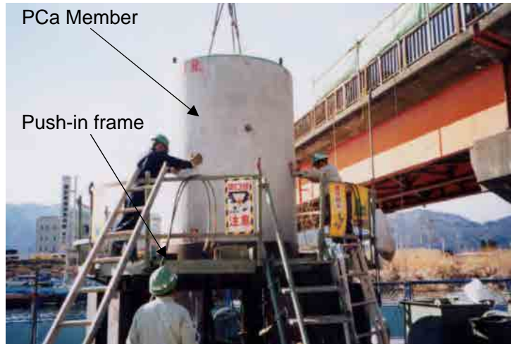
Figure 12-3-1. Installation of PCa member
