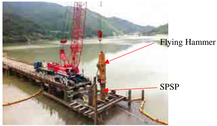
Figure 11-2-7. Flying Hammer Construction Method
