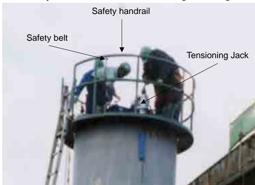
Figure 12-3-2. Tension work
