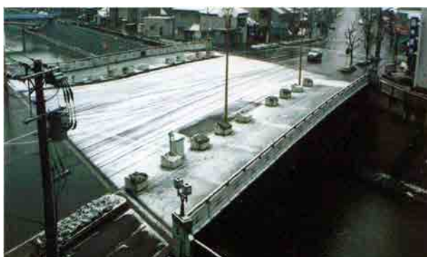
Figure 7-10-1. Freezing Status of Bridge Pavement Using Steel Deck
