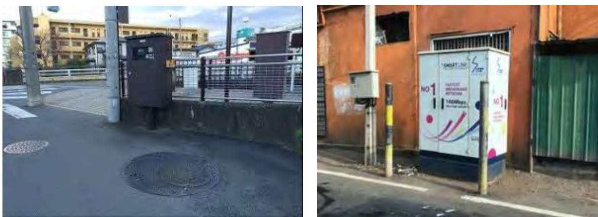
Figure 4.5-1 Power Supply Unit for Manhole-type Pump Stations and Telecommunication Services
