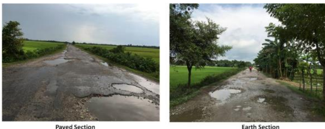
Figure 3-5: Present Conditions of Paved and Unpaved Sections
