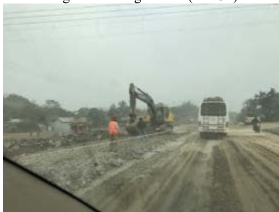
Road improvement and repair (NH-34)
