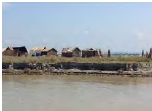
Erosion of the Char Land
