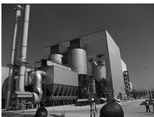
Rappi incineration plant with power generation
