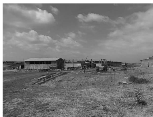
Bole transfer station (under construction)
