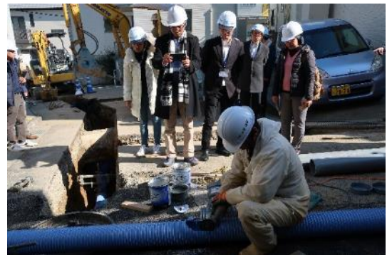
Construction site of a main sewer pipe
