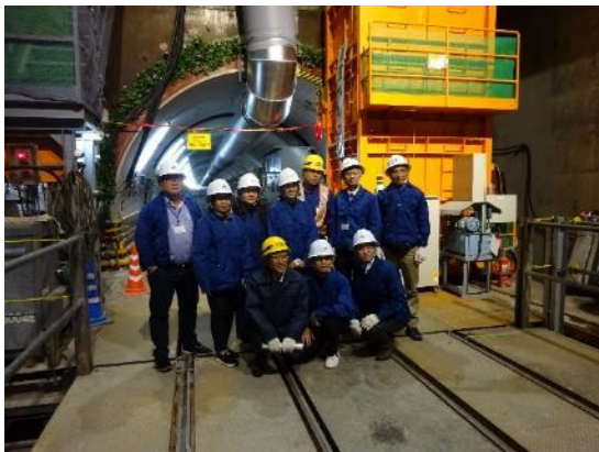
Starting shaft of rainwater storage pipe
