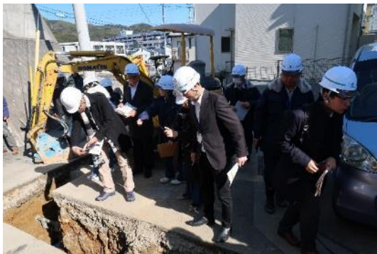
Construction site of a main sewer pipe
