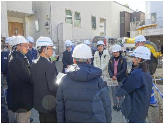
Construction site of house connection
