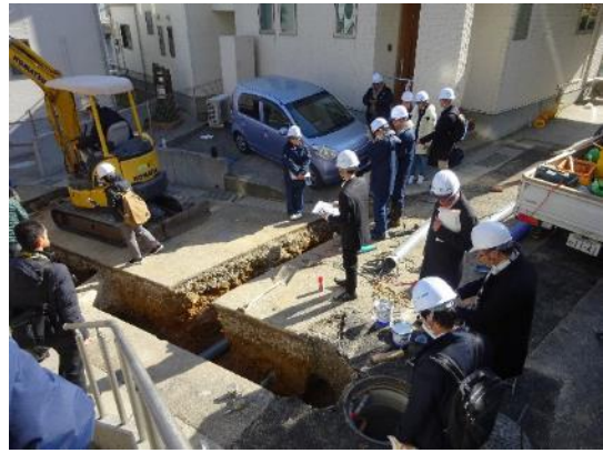
Construction site of a main sewer pipe
