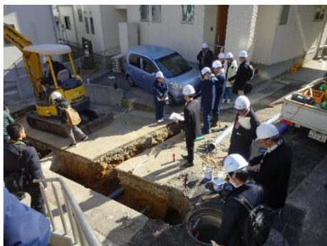
Construction site of a main sewer pipe
