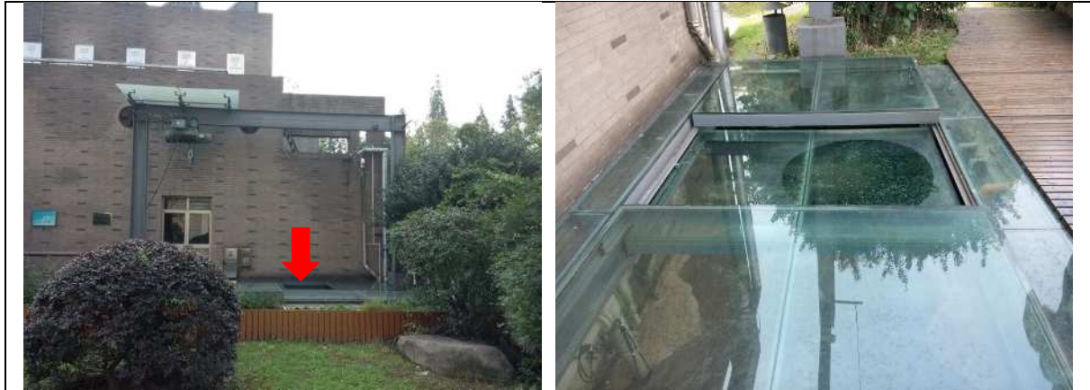
Figure 11.3.1 Example Case of Treatment Tank with Removable Strengthened Glass Covers
