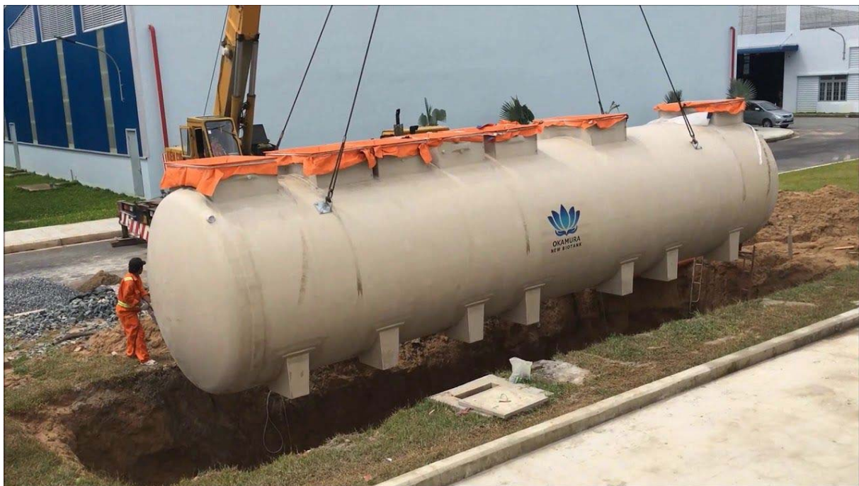
Figure.2 Example of the Structure of Medium-Scale Johkasou (FRP-made)
