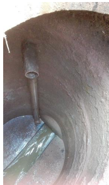
Inside of a manhole
