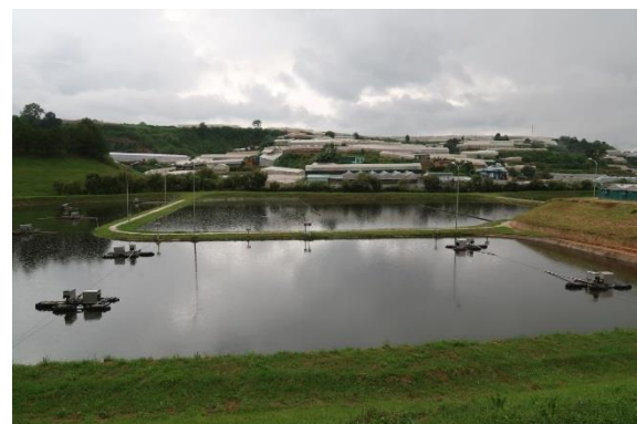
Aerated Lagoon (not used at present)
