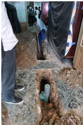
House connection work (inside of the house)
