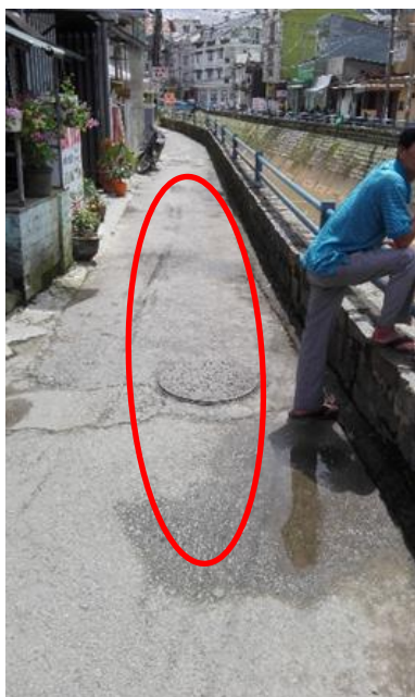
Pipe is installed along the river
