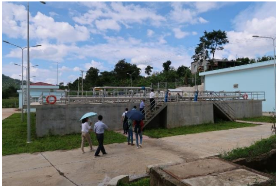
Outer side of treatment tank
