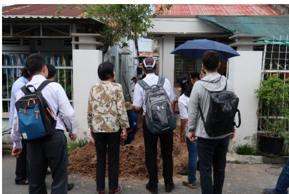
Figure 13 House connection work in Binh Duong province
