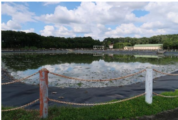
Anaerobic pond (A1, A2)
