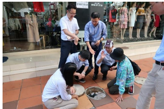
Checking of inside of connection box
