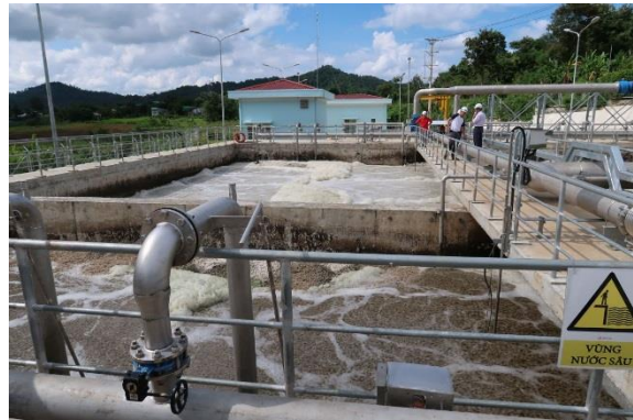
MBBR tank and sedimentation tank
