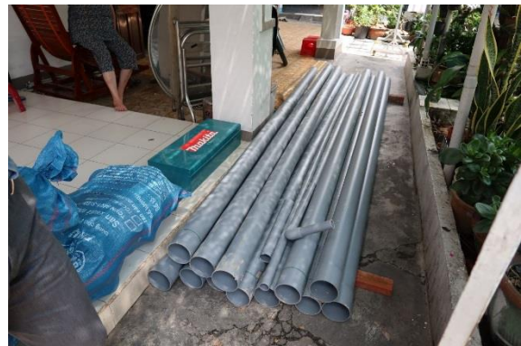
Pipes for house connection
