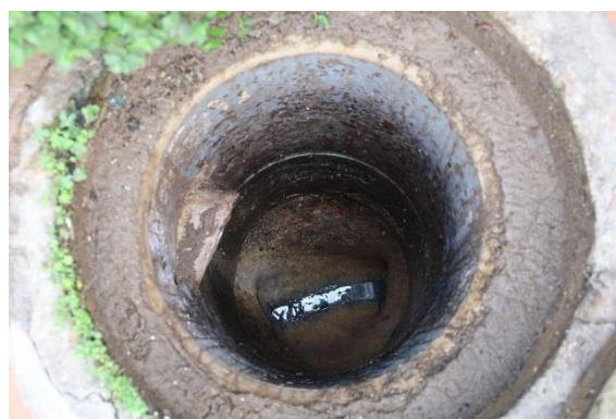
Inside of a manhole
