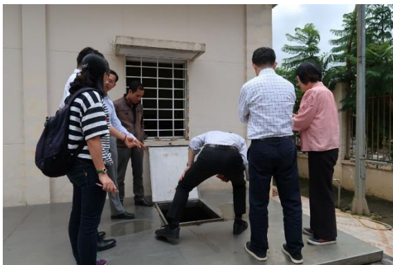
Checking of inside of pump pit
