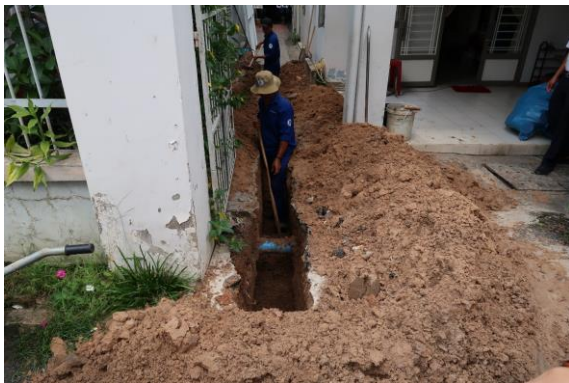
House connection work
