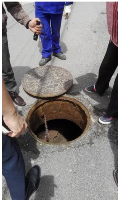
Inside of a manhole
