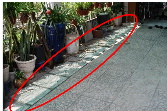
Tile is changed after the construction.
