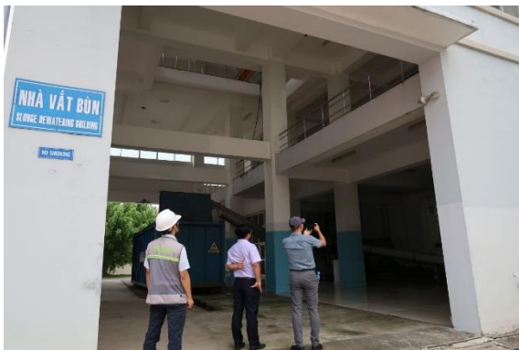
Sludge treatment building
