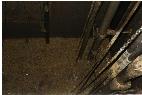
Inside of pump pit
