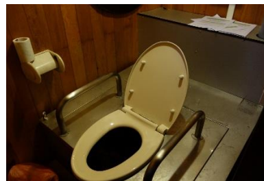
Composting Toilet Installed
