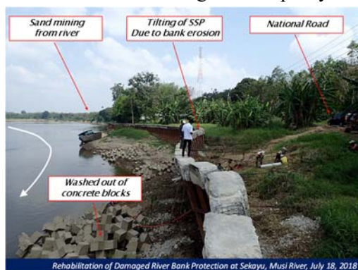
Figure G 9.1.1 Photo and Mechanism of River Bank Erosion at Sekayu
