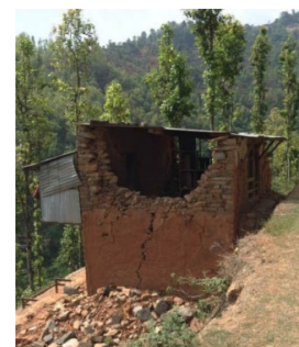
Fig. 7. Out-of-plane destruction in other country
