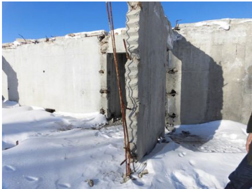
Fig. 12. Detail of vertical joint: Deconstruction building
