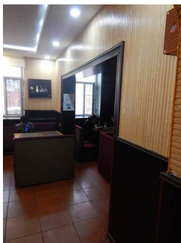
Figure 2. Masonry building where walls were removed for use as a store
