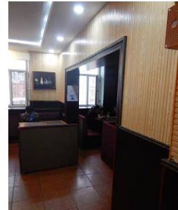
Fig. 4. Masonry building where walls were removed for use as a store
