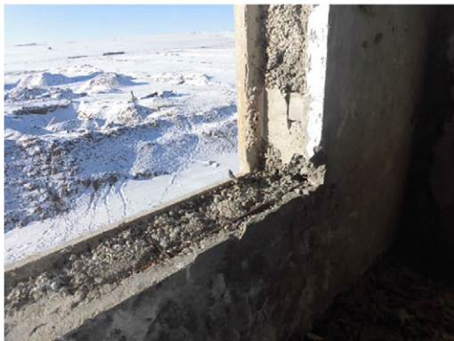
Fig. 13. Exterior wall with insulation layer: Deconstruction building
