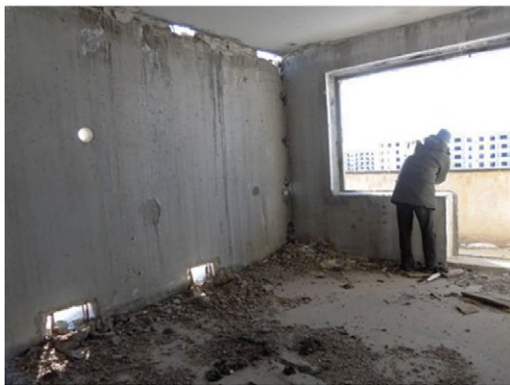
Fig. 11. Inner wall and exterior wall: Deconstruction building
