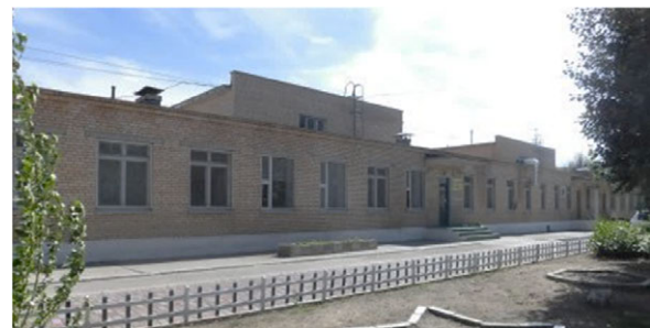
Fig. 2. Typical kindergarten building by masonry
