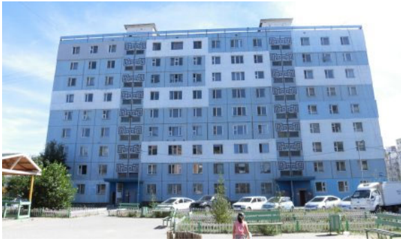
Fig. 3. Typical apartment house by precast panel structure
