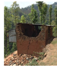
Figure 5 Out-of-plane destruction in other country
