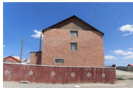
Fig. 6. Out-of-plane direction vulnerable building in Mongolia
