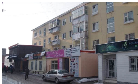
Figure 1. Masonry building first floor converted into stores
