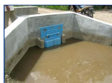
Photo 10.4.4 Gates on Secondary and Tertiary Canals
