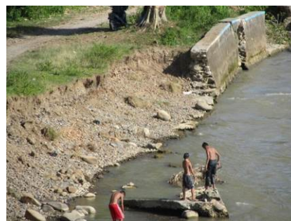
Existing retaining wall destroyed by flood in the Lematang River (027)
