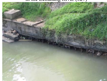
Insufficient foundation of revetment works in tributary of the Lematang River (024)
