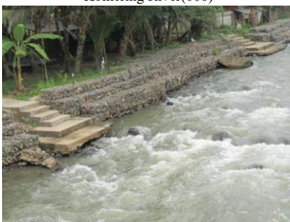
Subsidence and deformation of revetment works by erosion in tributary of the Lematang River (022)
