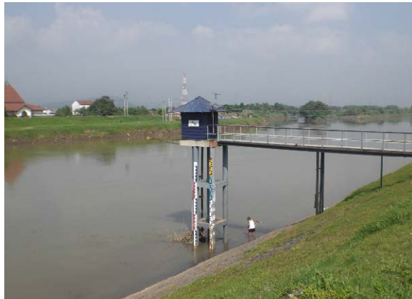
Porong Automatic Water Level Gauging Station
