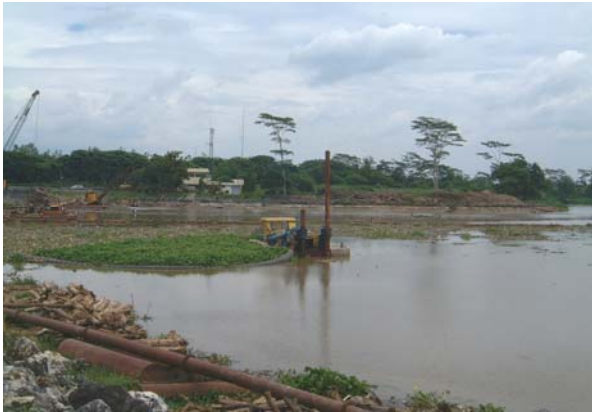
Sengguruh Dam (Maintenance Dredging in the Reservoir)
