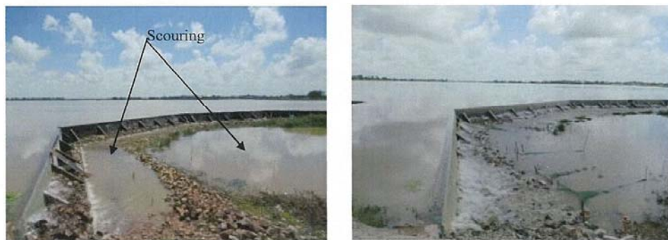
Figure A8-1 Vay Kor Dam During Placing Cobbles (Left) and After Placing Cobbles (Right) against Scouring in the Downstream Side of the Dam
