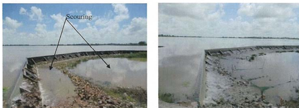
Figure A8-1 Vay Kor Dam During Placing Cobles (Left) and After Placing Cobles (Right) against Scouring in the Downstream Side of the Dam
