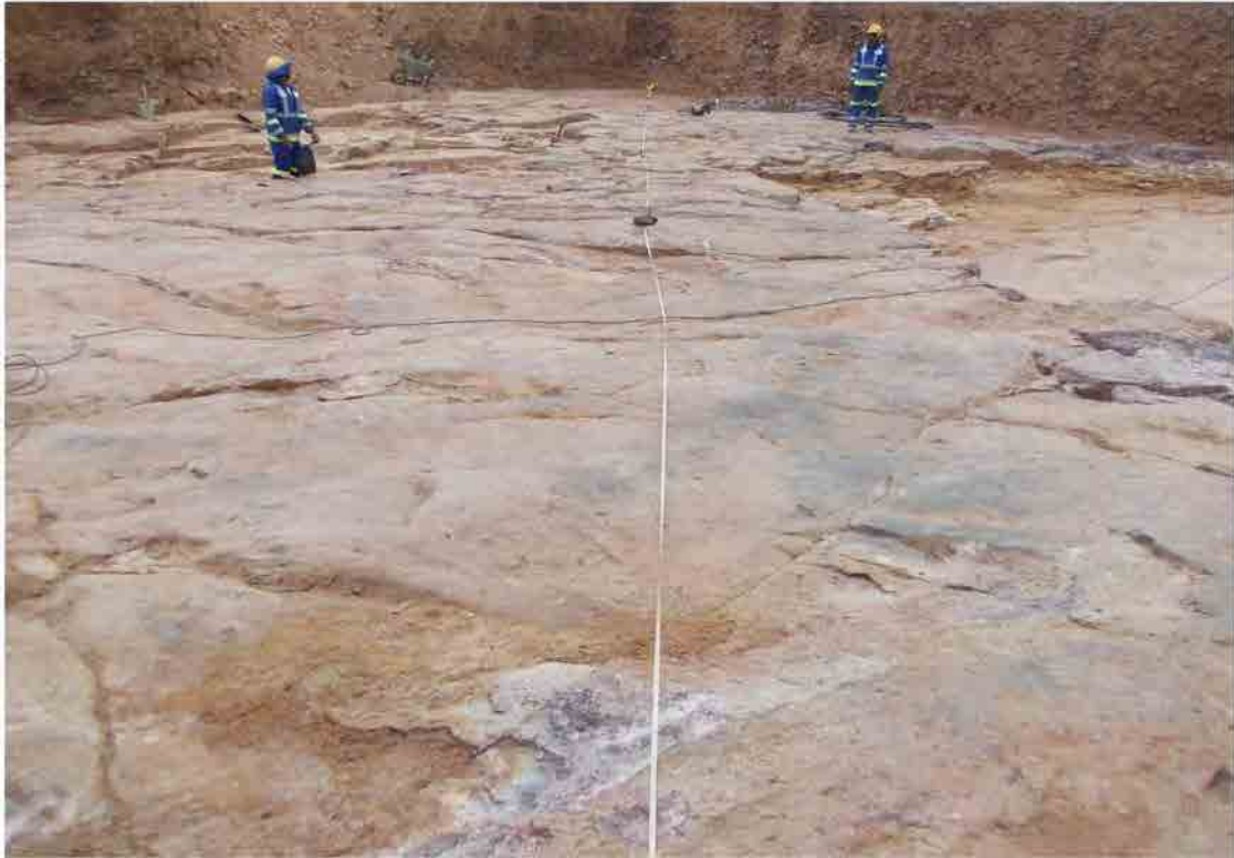
Figure 5.4-1 FGD Foundation Rock (Unit 2)
