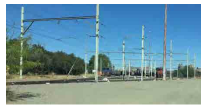
Railway Yard Owned by PPC
