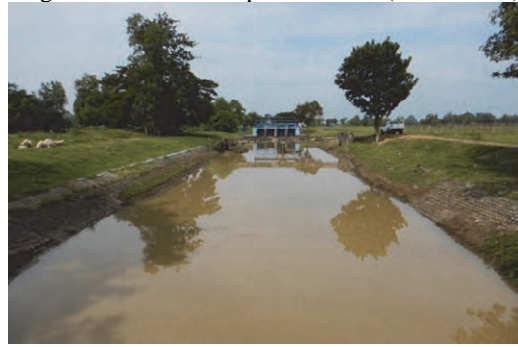
Irrigation Canal and Inspection Road (KM16+100)
