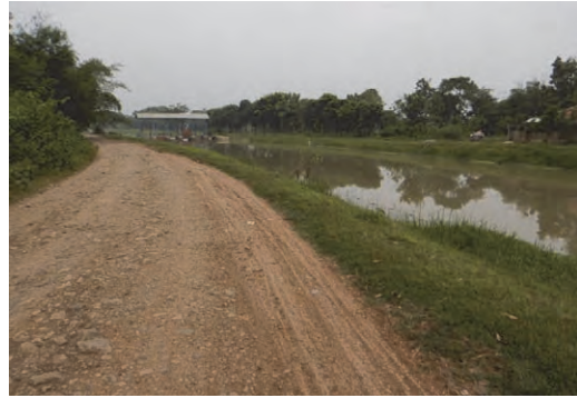
Irrigation Canal and Inspection Road (KM12+140)
