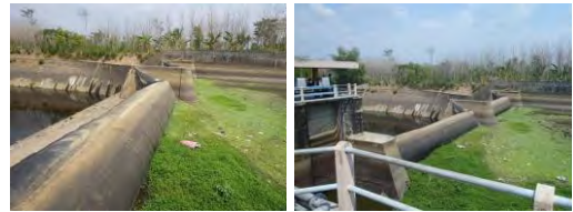
Doesn't functional away from half year ago. The rubber was damage and can't operated (replace ASAP)
