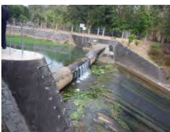
Original Bridgestone has Functional but only a few year to operation (must replace)
