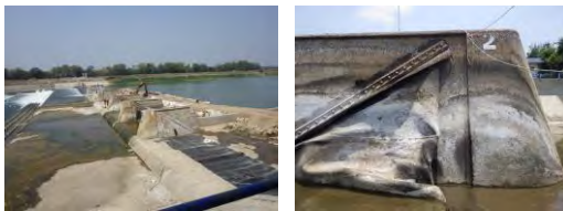
All span was replace to china product
