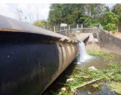
Original Bridgestone has Functional but only a few year to operation (must replace)
