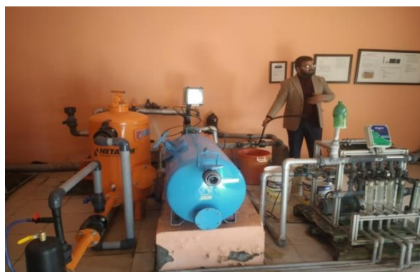
The Micro Irrigation System with Automation installed in the CoE of Sub-Tropical Fruits in Ladwa. (Kurukshetra district, 10 th February.2023)
