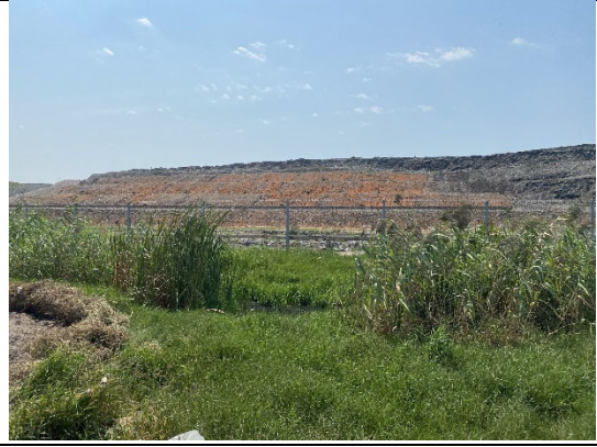
Visit to confirm the current status of Hulene dump site, 11 th
