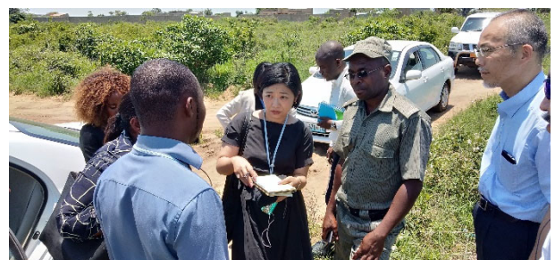
On-site visit of Mathlemele sanitary landfill construction site (28 th )
