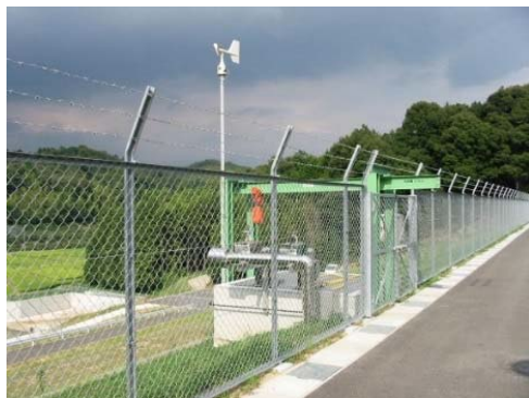
Example of anemometer installation
