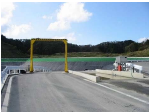
Example of water sprinkler system installation
