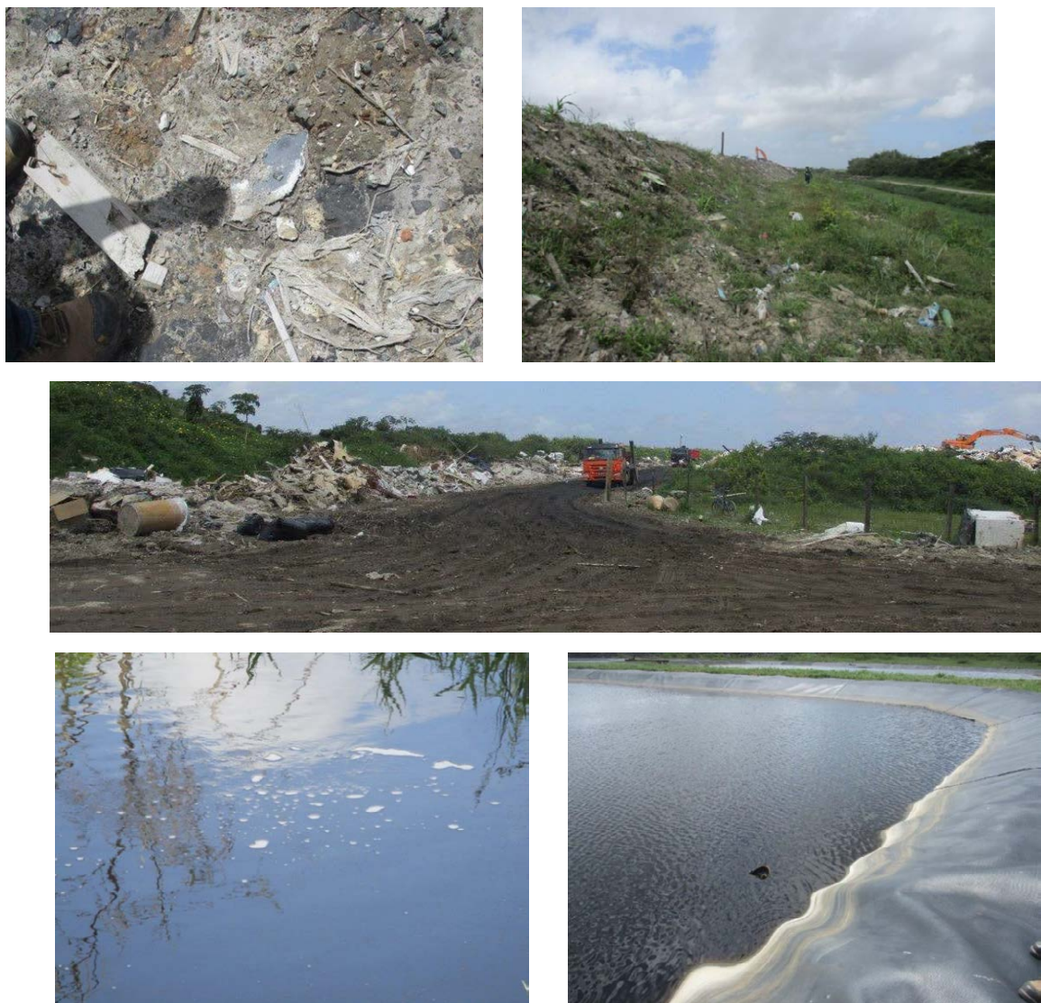
Figure 2-2: Haag Bosch Sanitary Landfill (top left: uncovered refuse surface layer, top right: small section of refuse layer 1, middle: Cell#2 loading dock, bottom: leachate treatment pond)
