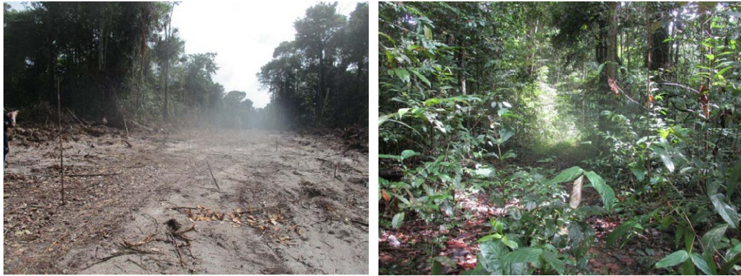
Figure 2-7: Bartica new landfill (left: access road, right: site entrance)
