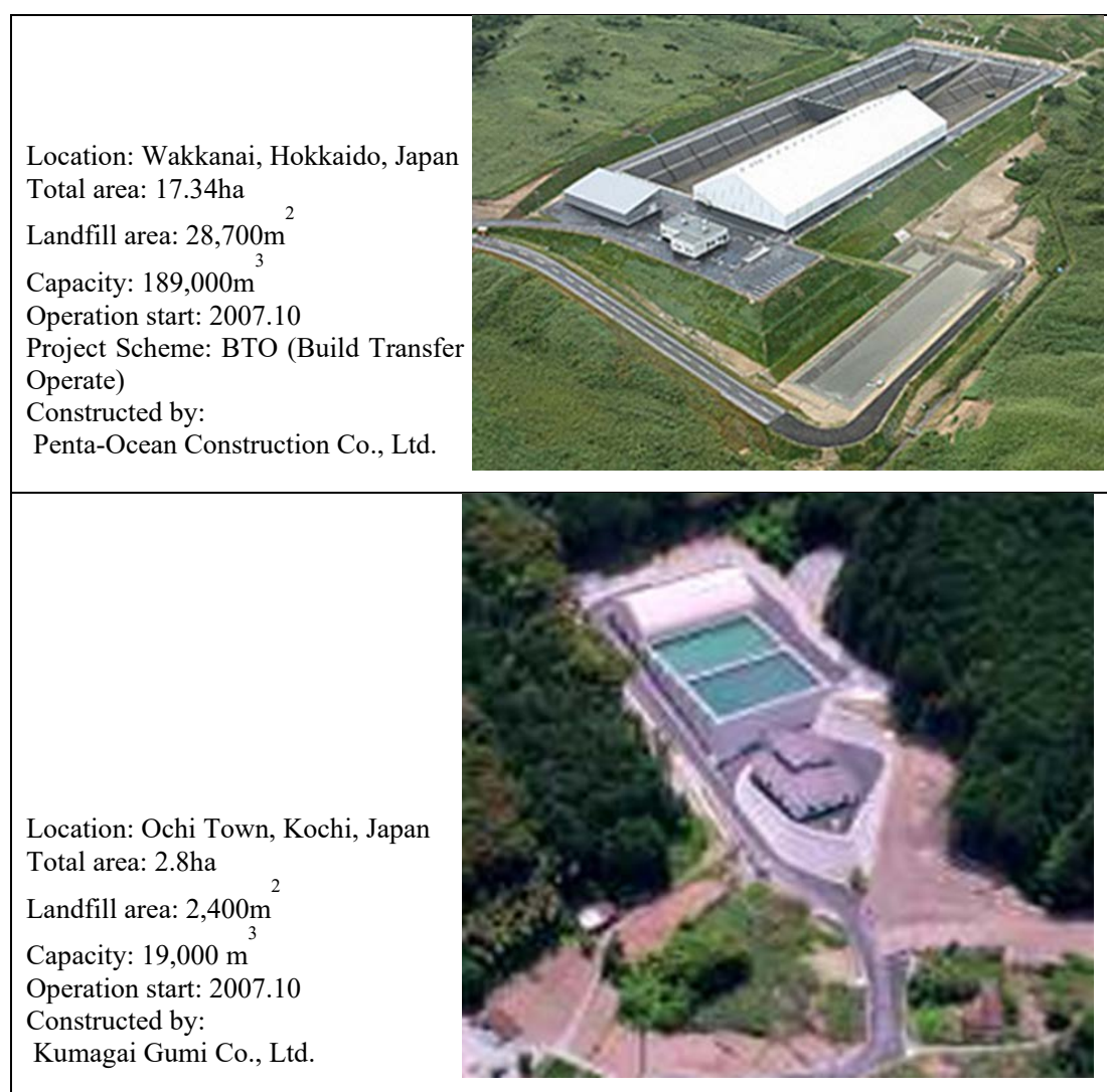
Figure 32: Examples of landfills with movable roofs
