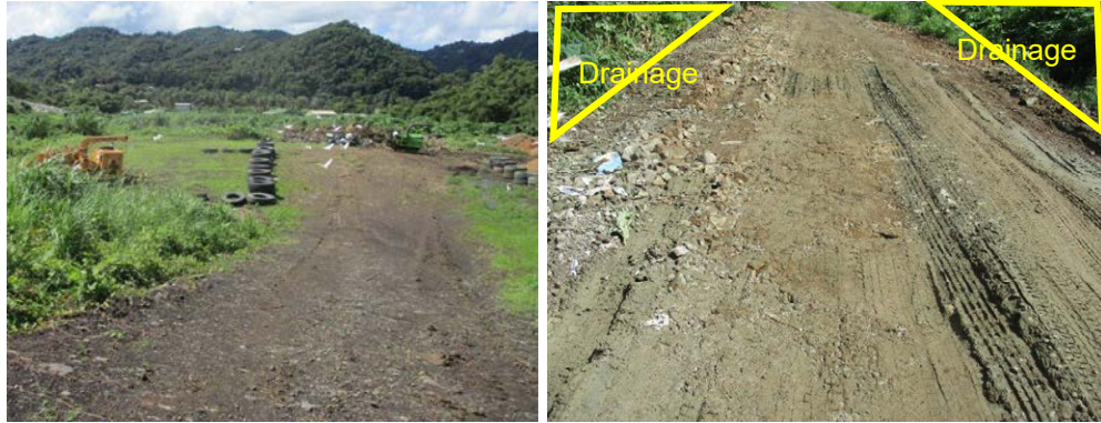
Figure 26: Good examples of drainage (Deglos Sanitary Landfill)
