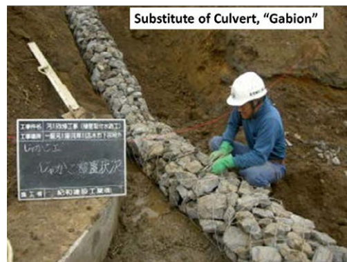
Figure 27: Gabion installation
