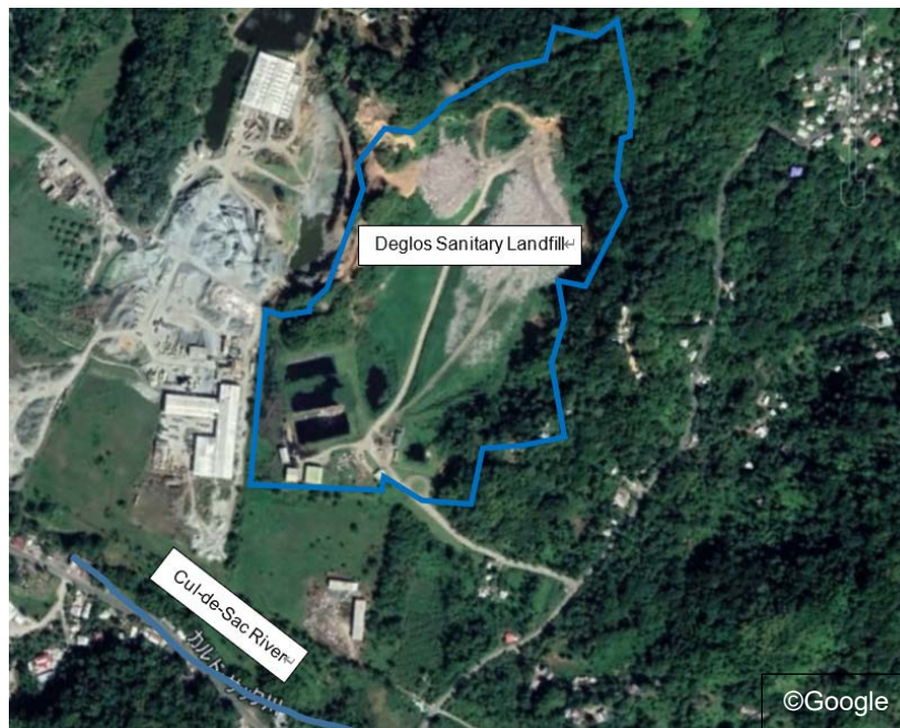
Figure 2: Deglos Sanitary Landfill (aerial photo)
