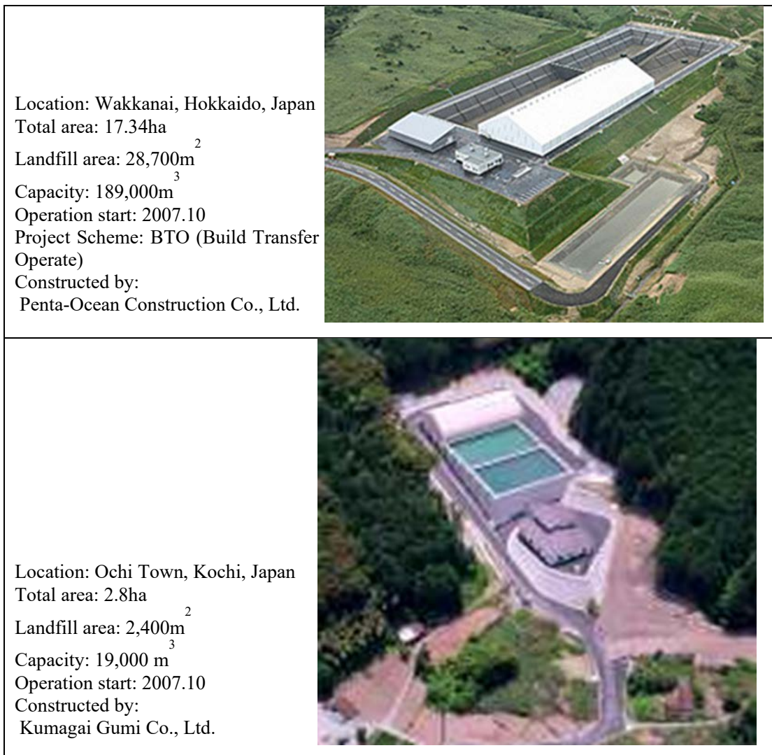
Figure 32: Examples of landfills with movable roofs
