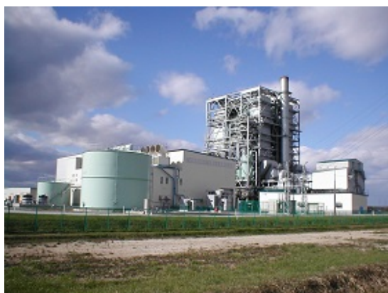
Panoramic view of Tomakomai Power Station
