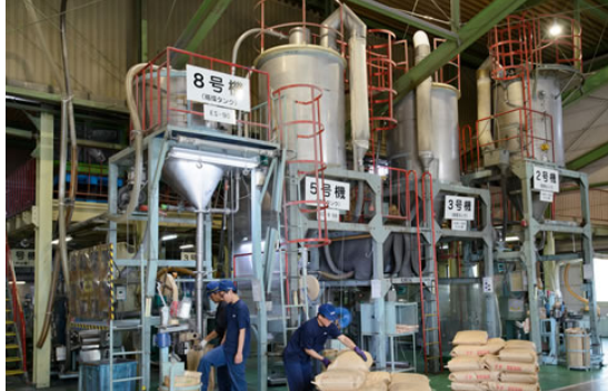
Stock tank with circulation function (silo)
