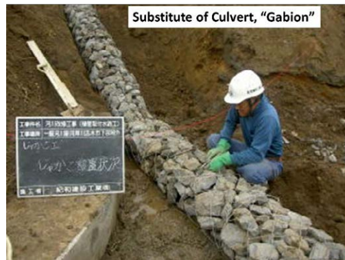
Figure 27: Gabion installation
