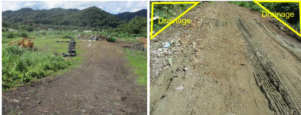
Figure 26: Good examples of drainage (Deglos Sanitary Landfill)
