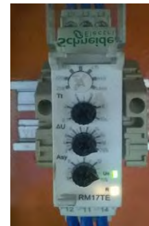
Phase Failure Relay
