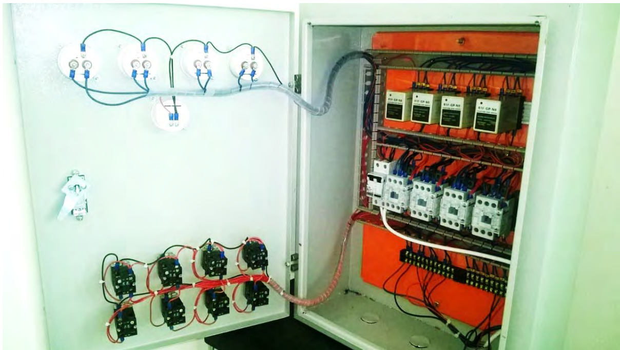
(DOL panel for miniature Pump Station)
