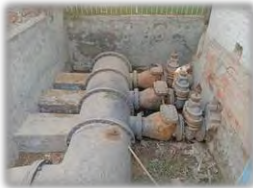
Discharge Valve & Check Valve
