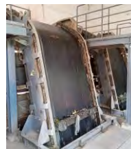
Bar Screen with Rake (Automatic)
