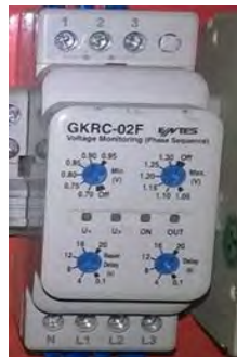
Under/Over Voltage Relay
