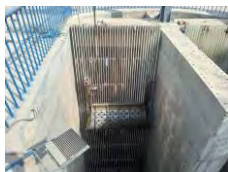
Bar Screen with Rake & Bucket (Automatic)
