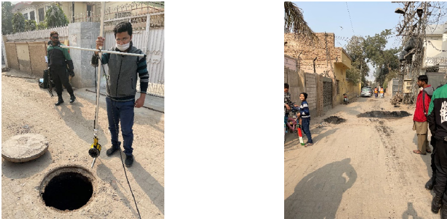
Picture 4.4.1 Demonstration of sewer camera at WASA-M and surrounding area
