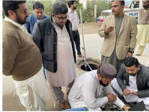
Photo 18: In-house training on analysis of inside sewer pipe by sewer camera
