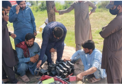
Photo 28: In-house training on butt fusion connection of HDPE pipes
