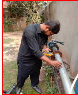
Thickness of Pipe wall
