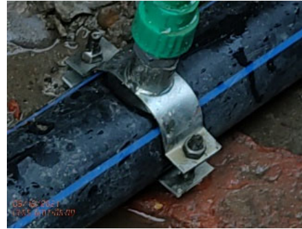
Connection of saddle to HDPE
