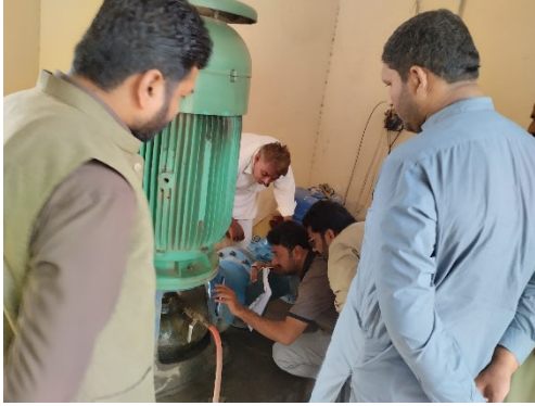
Photo 17: In-house training on O&M of pumps
