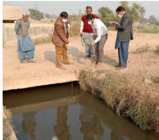
Measuring Right side of Drain
