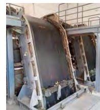
Bar Screen with Rake (Automatic)
