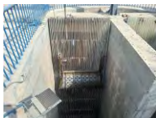
Bar Screen with Rake & Bucket (Automatic)
