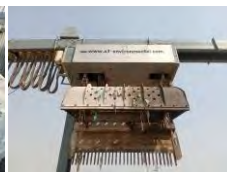
Bar Screen with Rake & Bucket (Automatic)
