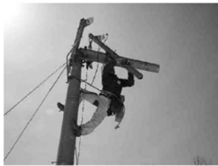
Emergency response to broken pole due to fallen tree (Actual site)
